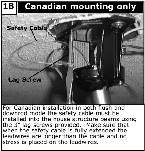
For Canadian installation in both flush and downrod mode the safety cable must be installed into the house structure beams using the 3" lag screws provided. Make sure that when the safety cable is fully extended the leadwires are longer than the cable and no stress is placed on the leadwires.
